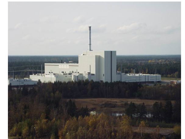
Figure 9.17 Forsmark 3 reactor - 3157 MW thermal power
