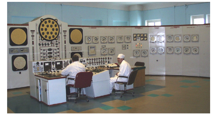
Figure 1.54 The control room of the Obninsk reactor.
