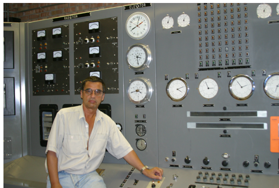
Figure 1.50 The control panel of the EBR-1
